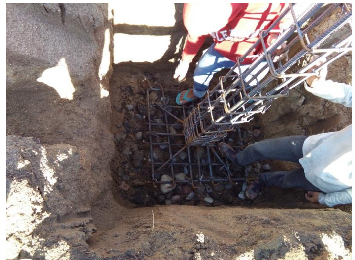
Excavation and installation of footings and columns reinforcement on November 8, 2018
