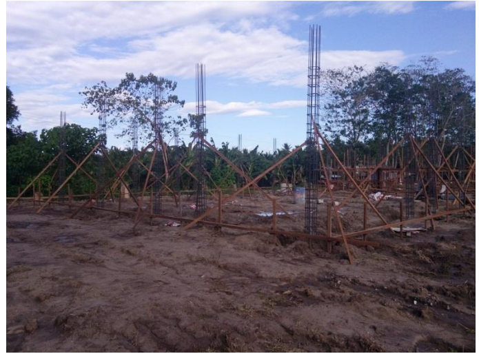
Installation of forms and reinforcement of column installed on November 8, 2018
