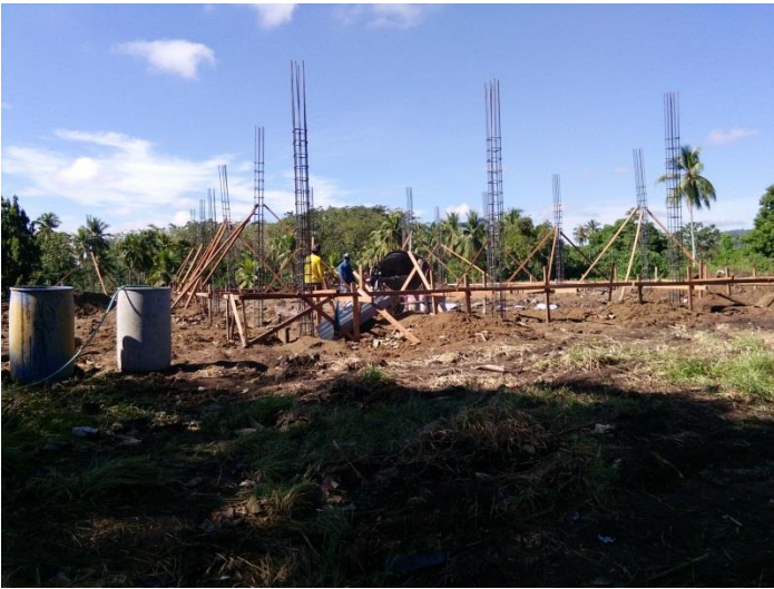
Installation of forms and reinforcement of column installed on November 8, 2018
