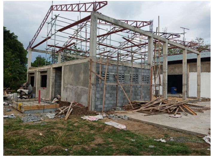
Installation of steel trusses on March 27, 2019
