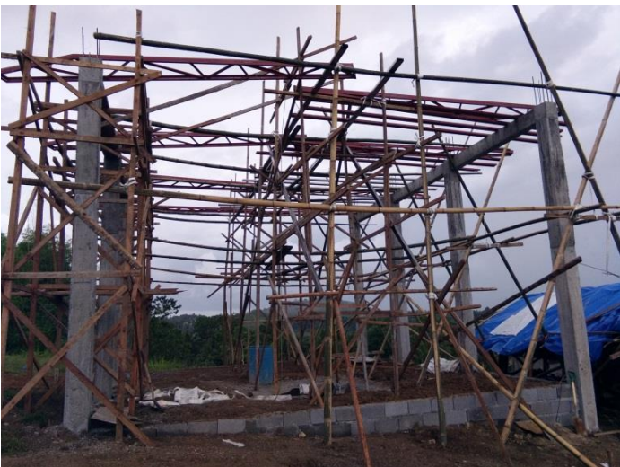
Installation of steel trusses on August 18, 2017
