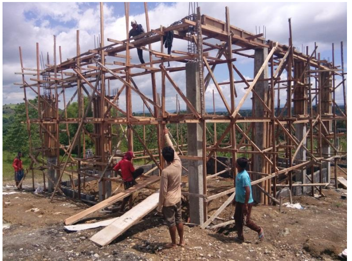
Pouring of concrete on column and roof beam
