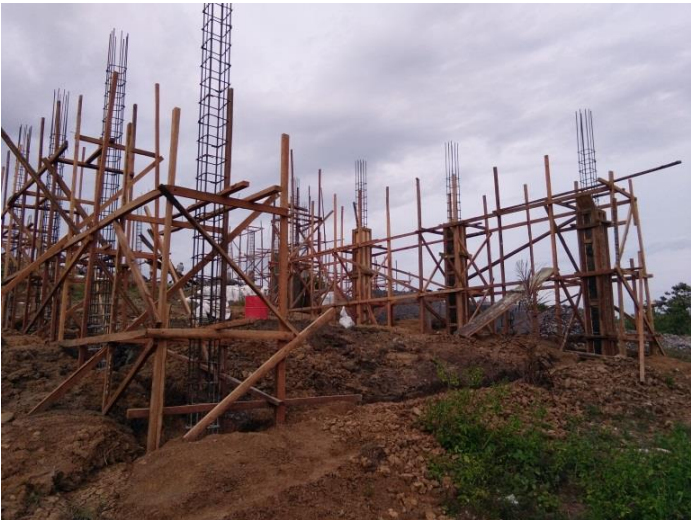
Installation of Column forms and reinforcement
