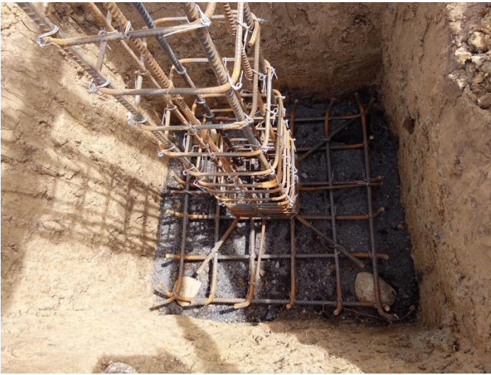
Installation of Footing and Column reinforcement
