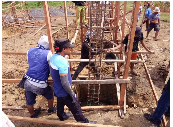
Pouring of concrete on footing on July 28, 2019
